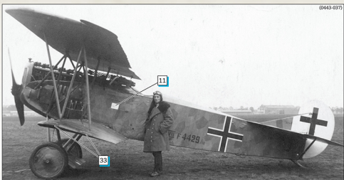
Fokker D.VII F 4429/18 makes for an imposing backdrop to this photograph of a young unidentified pilot. Note the Fokker style of wing tip handling instructions (33), rigging/assembly instructions (11) doped to the side of the 4 colour lozenge fabric covered fuselage and height of the LMG 08/15 'Spandau' machine guns. Göring's Fokker D.VII F 5125/18 would have appeared very similar to this before being overpainted white at the factory.
